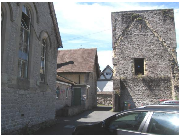
Scout building (left) and Priory (right). One end of the LF doublet passed right over the Priory, thanks to Chris's fishing rod skills.
